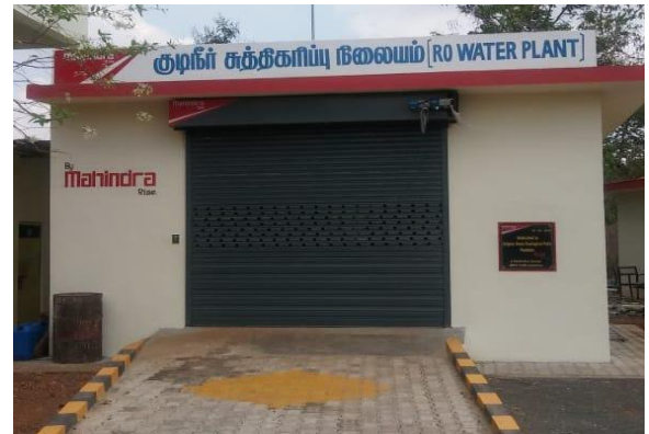
Centralized RO Unit (CSR Sponsored)
