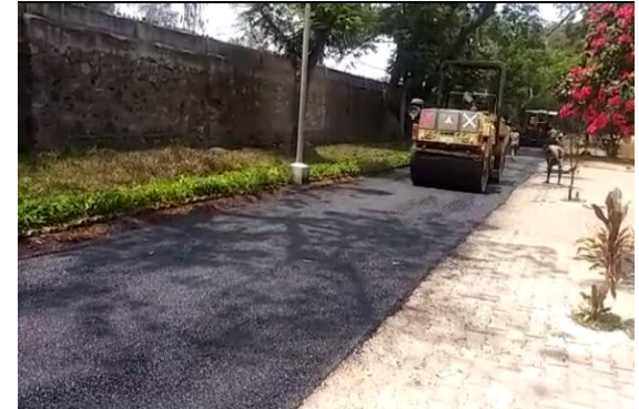
Black topping of Roads
